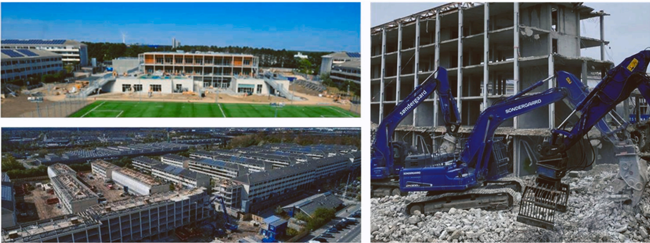
Fig. 1. View of the Taastrupgaard social housing area with approximately 1000 housing units, highlighting the demolition of eight apartment buildings that were recycled in the construction of the new city hall.
