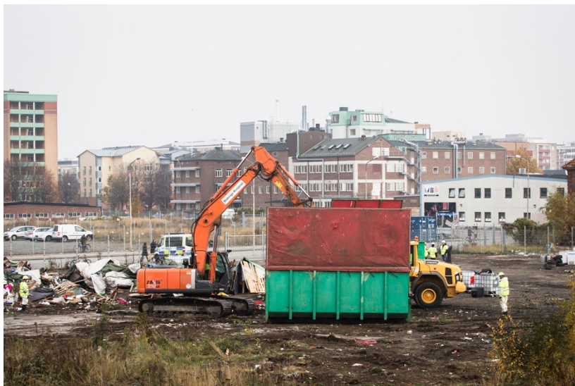
Figure 9. Wrecking crews demolishing the Sorgenfri camp. © Jenny Eliasson / Malmo Museums
