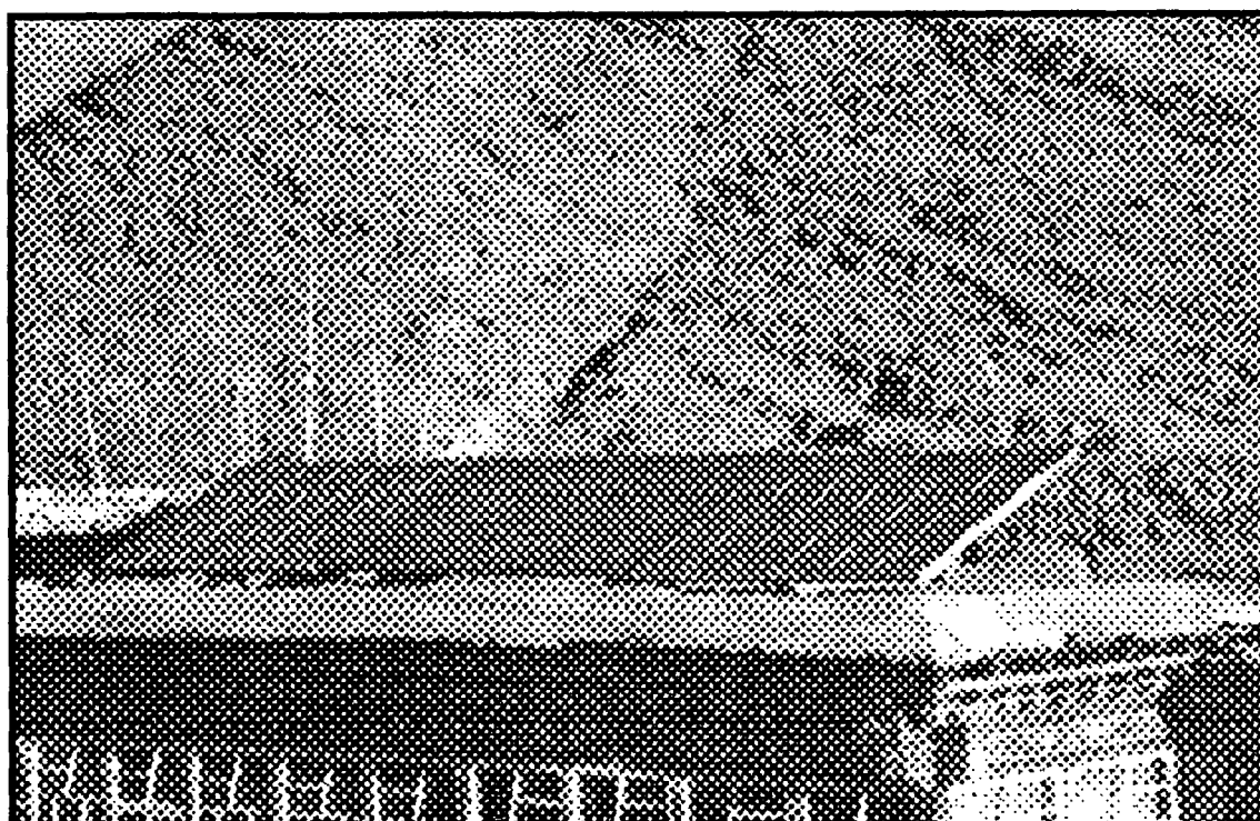
Figur 20. 2 kW fotovoltaisk installation i Lhasa, Tibet. (fra Sixth Research Institute, Tibet Solar Energy Research Institute).
