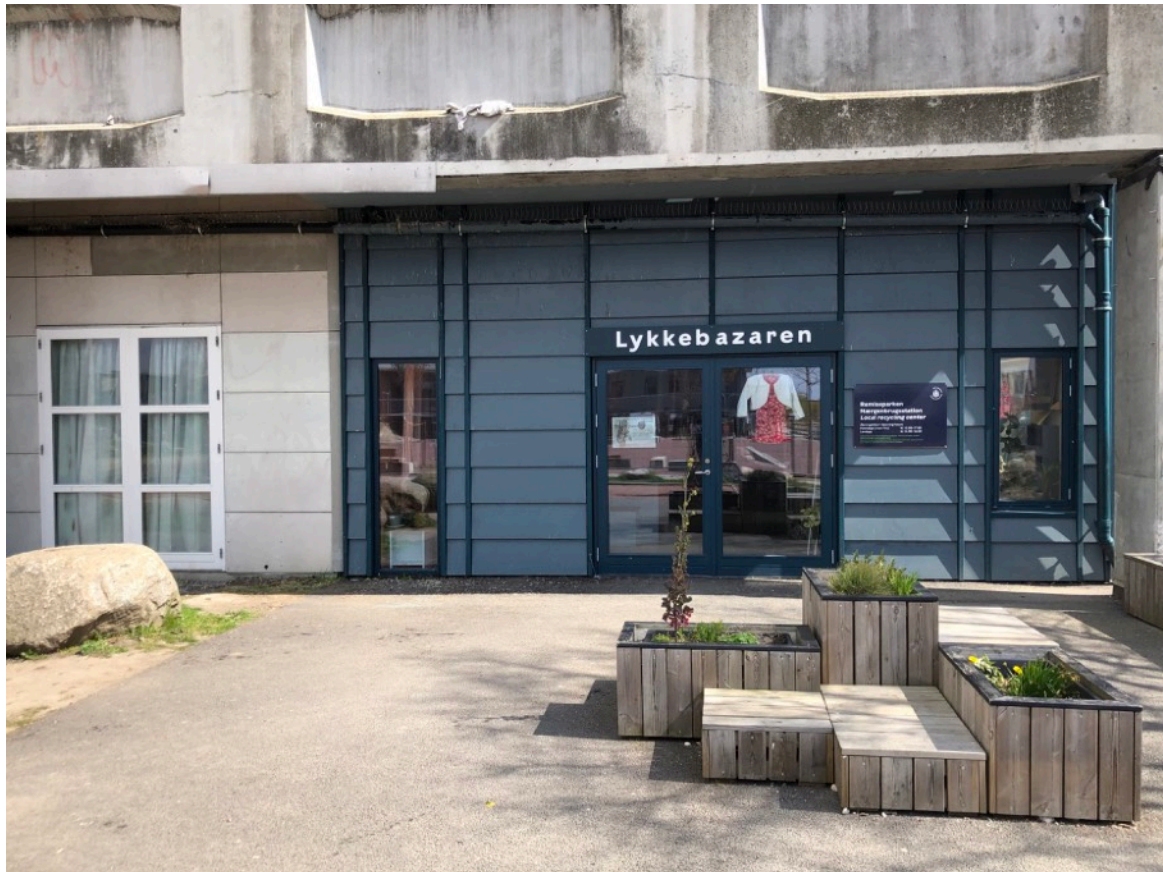
Redesigned facade slabs in Remiseparken
