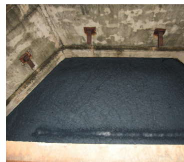
Wastewater of the company is treated in a microbiological tank
