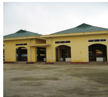
The new buildings financed by the project at Nông Trang market
