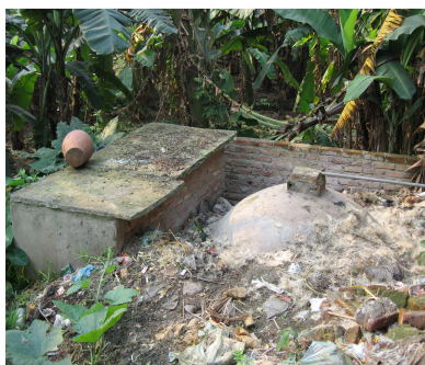
The tomb of a biogas plant (like others) is constructed under the earth
