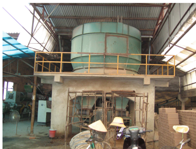
The grinder seen from the front side
