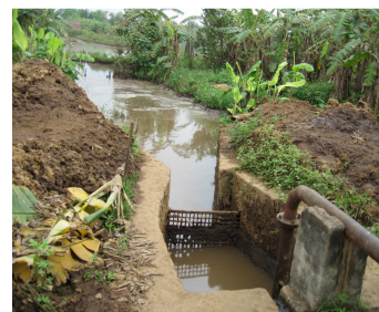
The reservoir where all the wastewater is gathered and receives preliminary treatment
