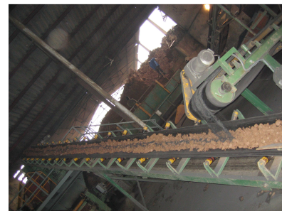
The redundant soil is being exploited by the grinder
