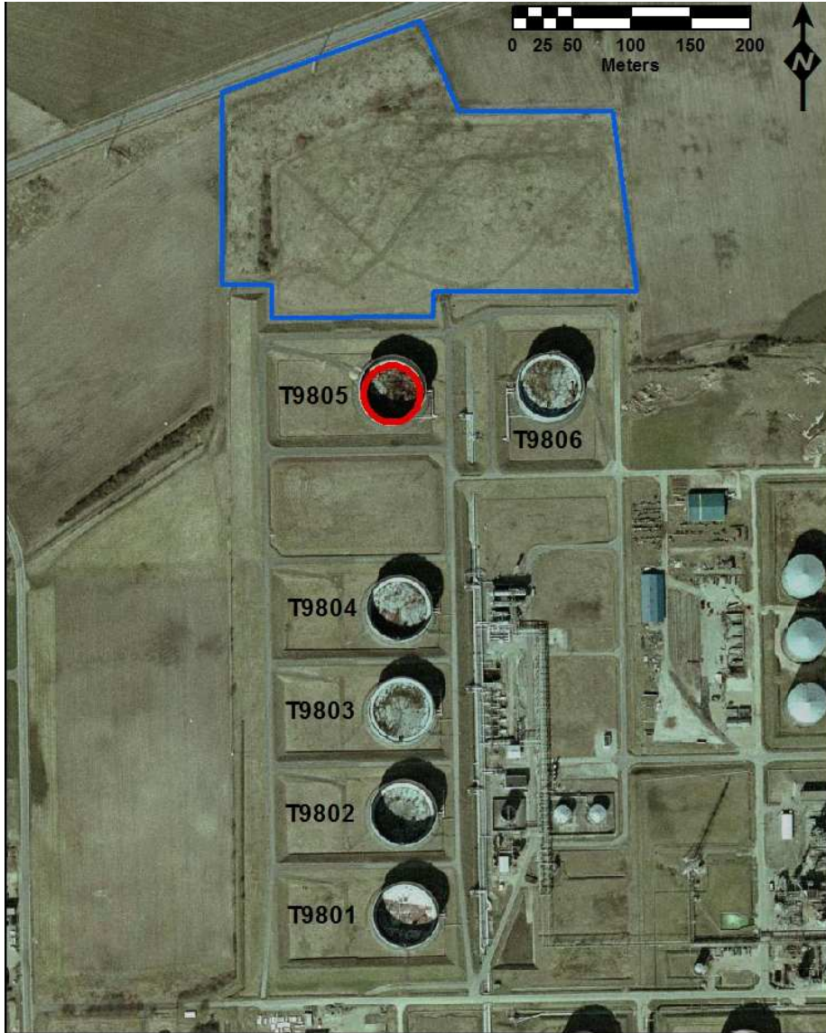
Figure 5.8: Orthophoto of the Fredericia oil terminal(Source: KMS). The numbers of the individual tanks are written in black. The tank studied in this project is marked with red. The area where the measurements are to be taken is marked with blue.
