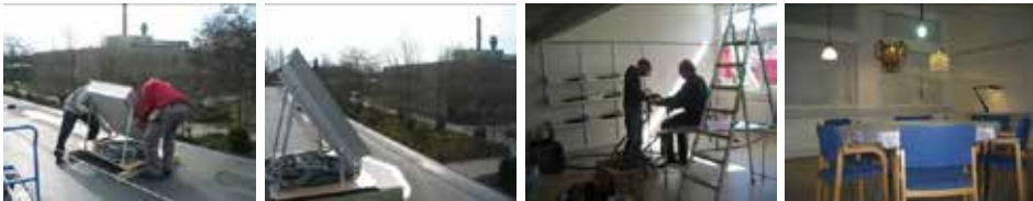
Picture 4, 5, 6, 7; from left to right: installation of the sol collector, installation of the optical fibers, installation of the luminaries, and disposition of the room.
