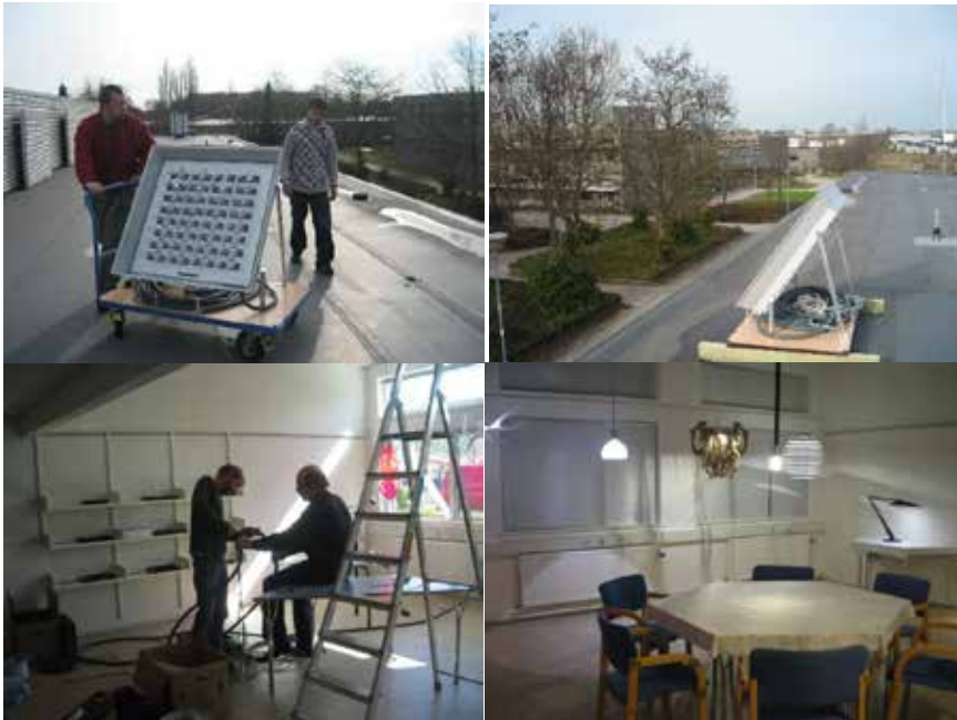
Pictures 7, 8, 9 and 10 From left to right: installation of the solar collector, installation of the optical fibres, and installation of the luminaires and the layout of the room.
