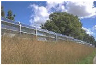
Figure 3 (left). PV panels mounted on road protection barrier at Fløng (NESA, built 1999).
